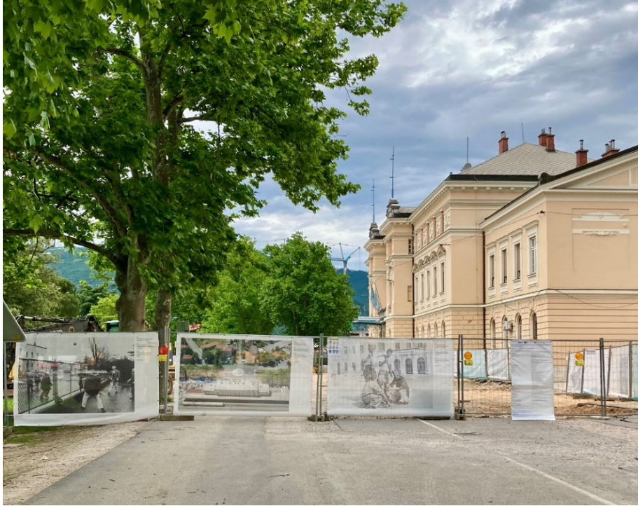
The Piazza Transalpina-Trg Evrope and the Transalpine railway station, currently under works in view of Nova Gorica-Gorizia's joint title as European Capital of Culture 2025. (26.05.2024)
