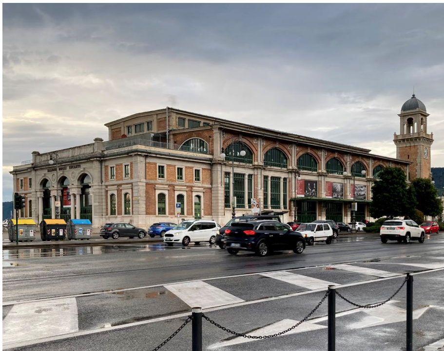
The Salone degli Incanti, expositive centre of Modern and contemporary art, formerly Trieste's central fishery. (31.05.2024)
